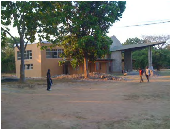
Two views of the JMTUC Chapel nearing completion.
